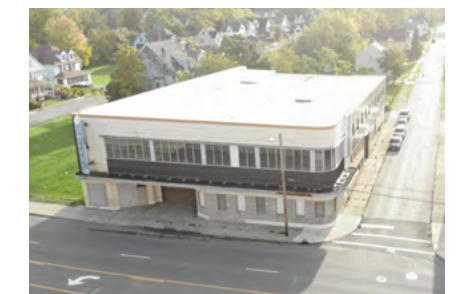
Aerial view of the Mickey's building before renovation.
