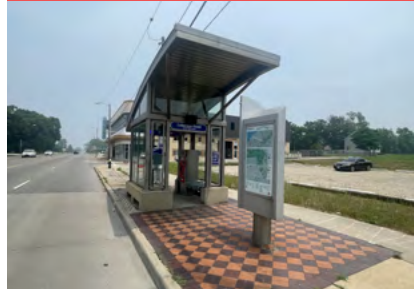
HealthLine BRT station in Circle East District.
