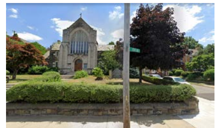
Image: Saint Philomena Church on Euclid Avenue in East Cleveland, Google 2022
